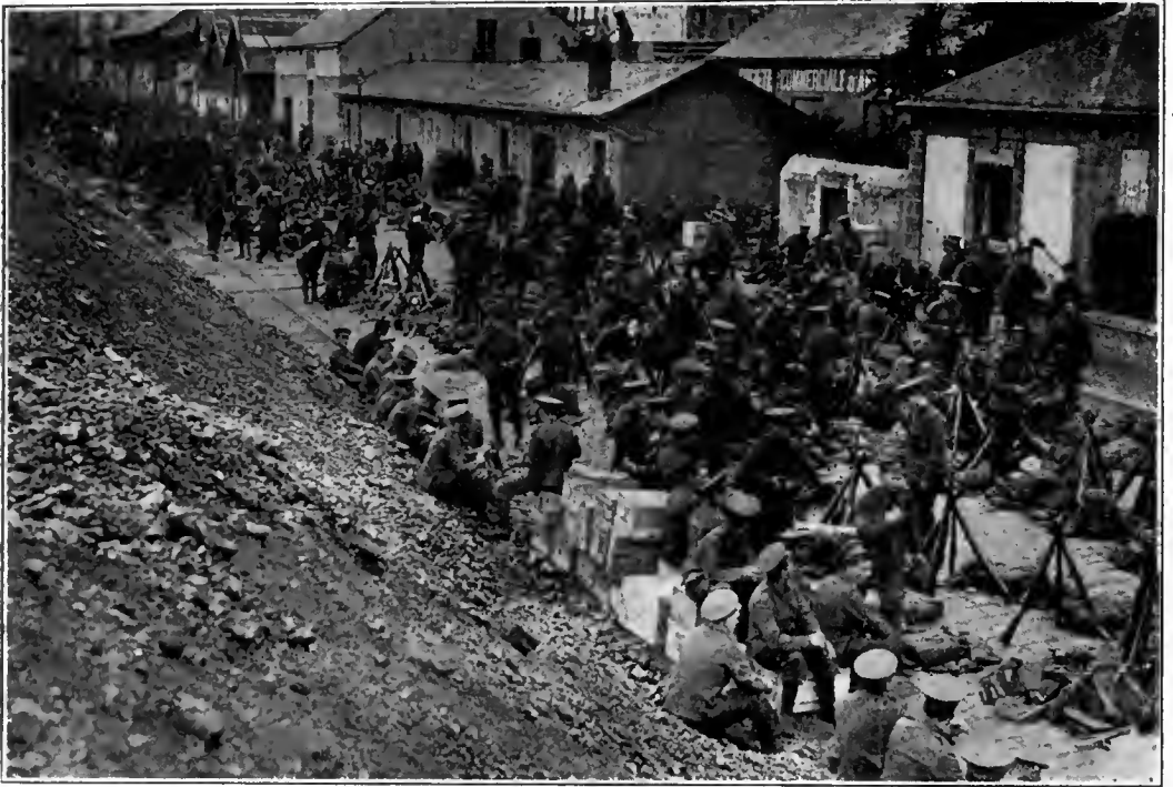
A BRITISH COLUMN HALTS BY THE WAY.
